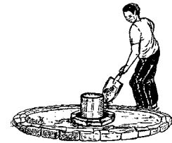
Pour the concrete slab and form the protective collar
