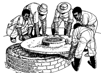
Set the cured well cover in place
