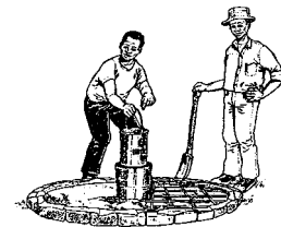
Place reinforcing wire and a mold for the hole
